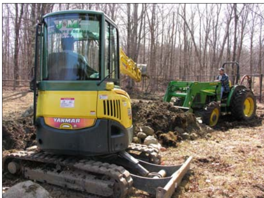
Excavation of the new pond begins.
