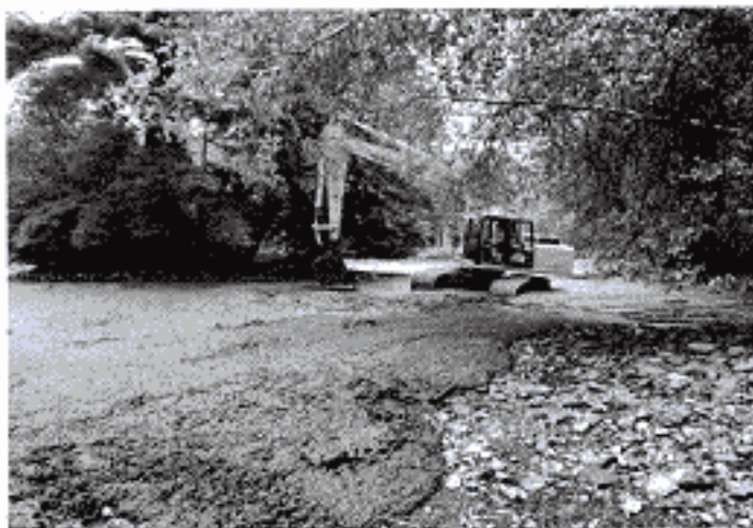
Dredging the large pond.
