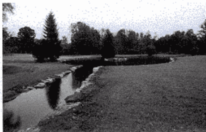
Canal pond completed.
