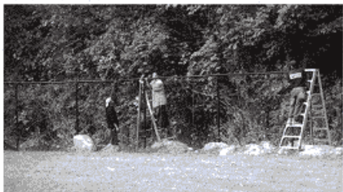
New perimeter fence
