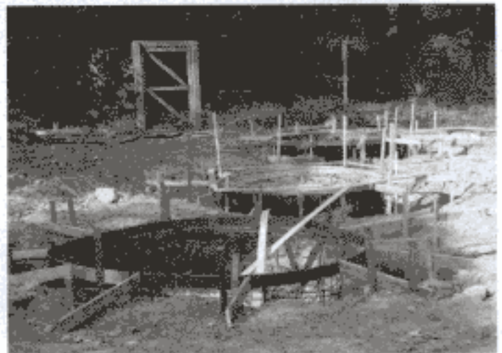
New breeding pens under construction
